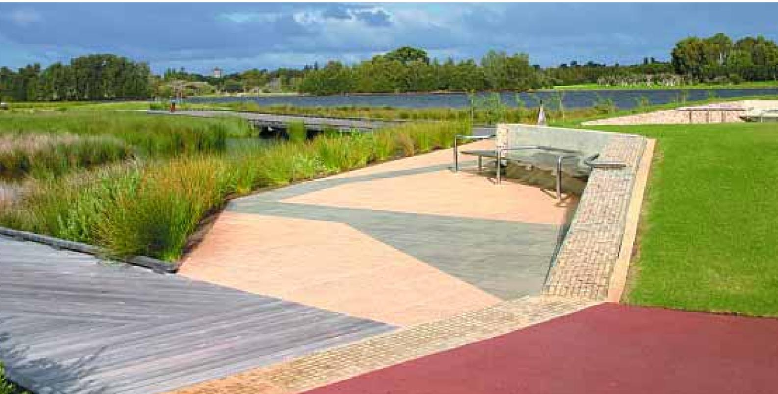
A series of folds, acting as transpiration swales, gives form to the Point Fraser Wetland. Endemic reeds and sedges are mass-planted throughout the bio-filter that cleans dirty stormwater runoff before discharge into the Swan River.
