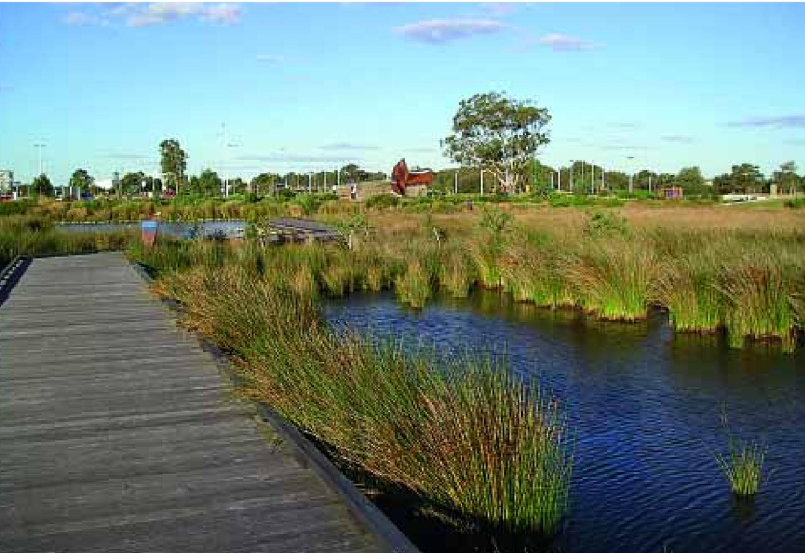
Boardwalks lead out over the bio-filter; a natural filtration system that significantly reduces nitrogen, phosphorus and sediment levels by moving polluted water through a series of highly engineered ponds planted with reeds and sedges. Man-made beaches for anchoring boats and canoes, are slotted between the swales.
