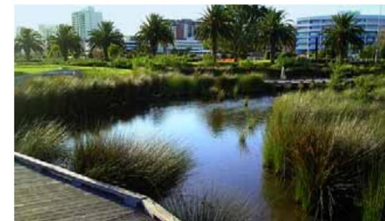
Zone aerates out-flowing water. Water entering the river after passing through the bio-filter is now at least 25 per cent less in nitrogen, 45 per cent less in phosphorous, and records a 75 per cent sediment reduction. Water exiting the bio-filter is now cleaner than the surrounding river water.
