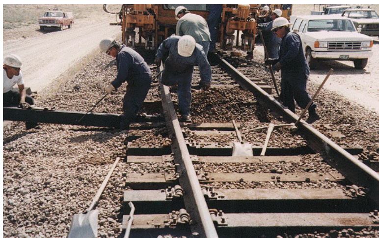
Figure 6. Recycled-plastic RR cross-ties being installed at test track in Pueblo, CO.
