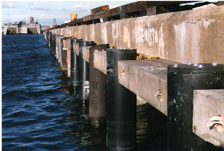
Figure 5. Recycled plastic pilings installed at Port Newark.
