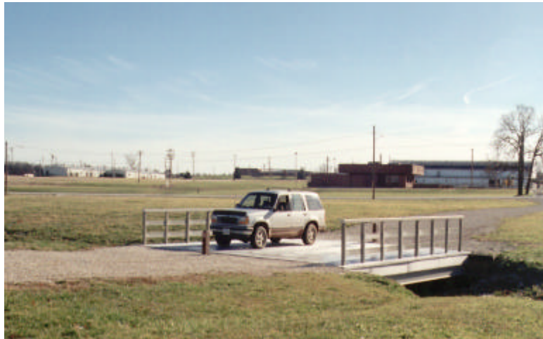
Figure 2. Sport utility vehicle driving over RPL bridge.
