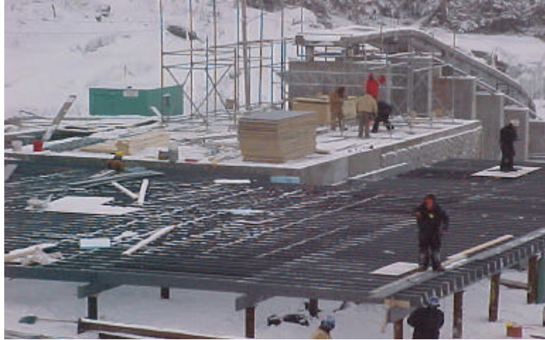
Figure 4. RPL platforms being constructed at Lake Placid.
